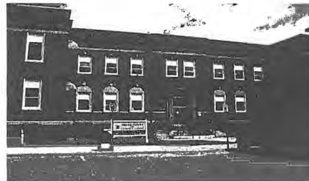
Bernadette Building (#48) Minimum and Work Release Unit
